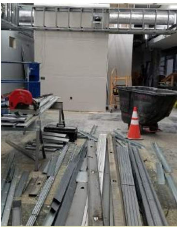
Building Under Construction
